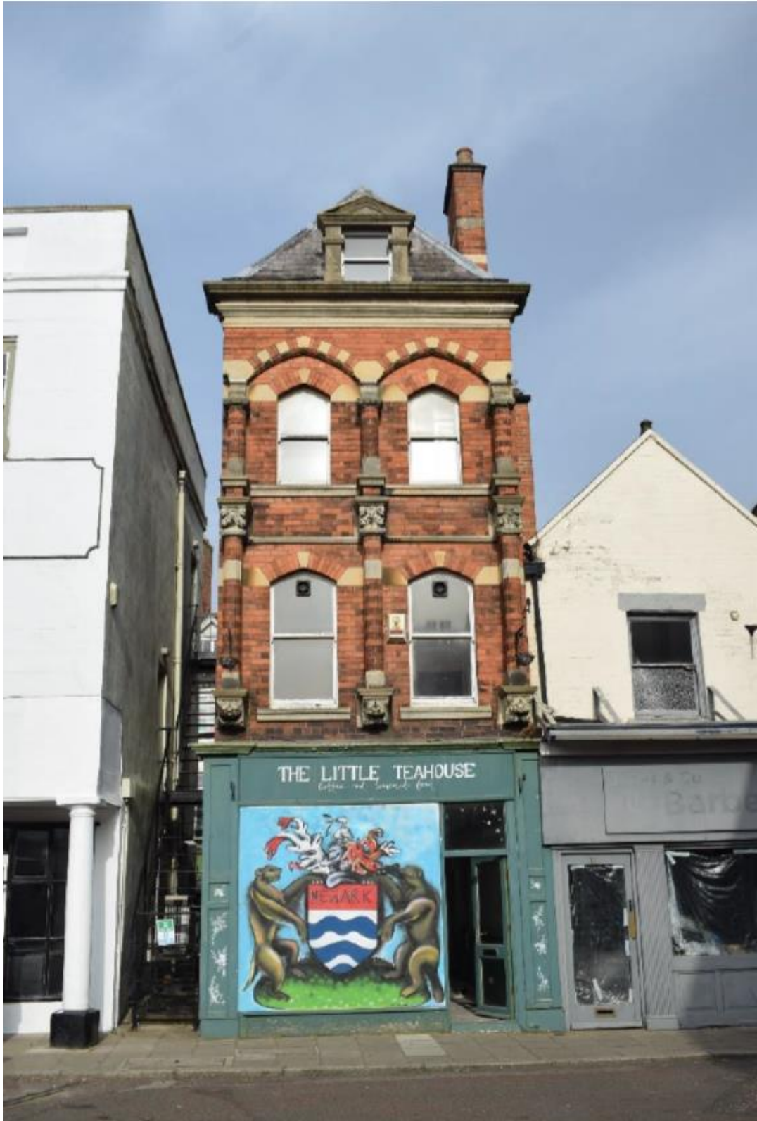
Front Elevation of 14 Market Place
