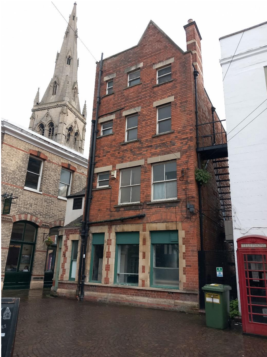
Rear Elevation of 14 Market Place
